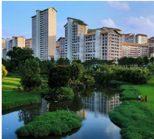
The naturalising of a concrete canal in Bishan-Ang Mo Kio Park through the Active, Beautiful and Clean (ABC) Waters programme.
