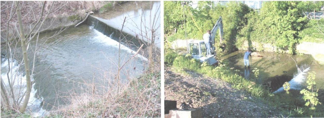
Weir built in the 1950s and representing an obstacle to fish migration in the river „Lauter”. Initial state before the implementation of the compensation measure in 2008. (Source: StadtLandFluss, internal documents).
