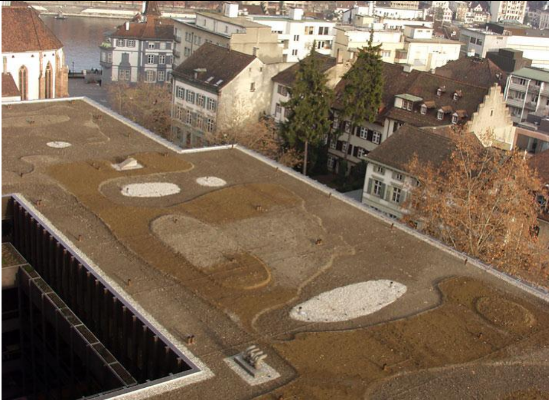
Figure 4. Newly constructed green roof on the Klinikum 2 of the Cantonal Hospital of Basel, built in accordance with the city's new guidelines on green roofs and urban biodiversity. Source: Brenneisen (2006).
